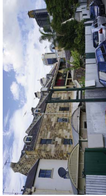
Fig. 34: Rear facades to Kent Street west, viewed from High Lane.
